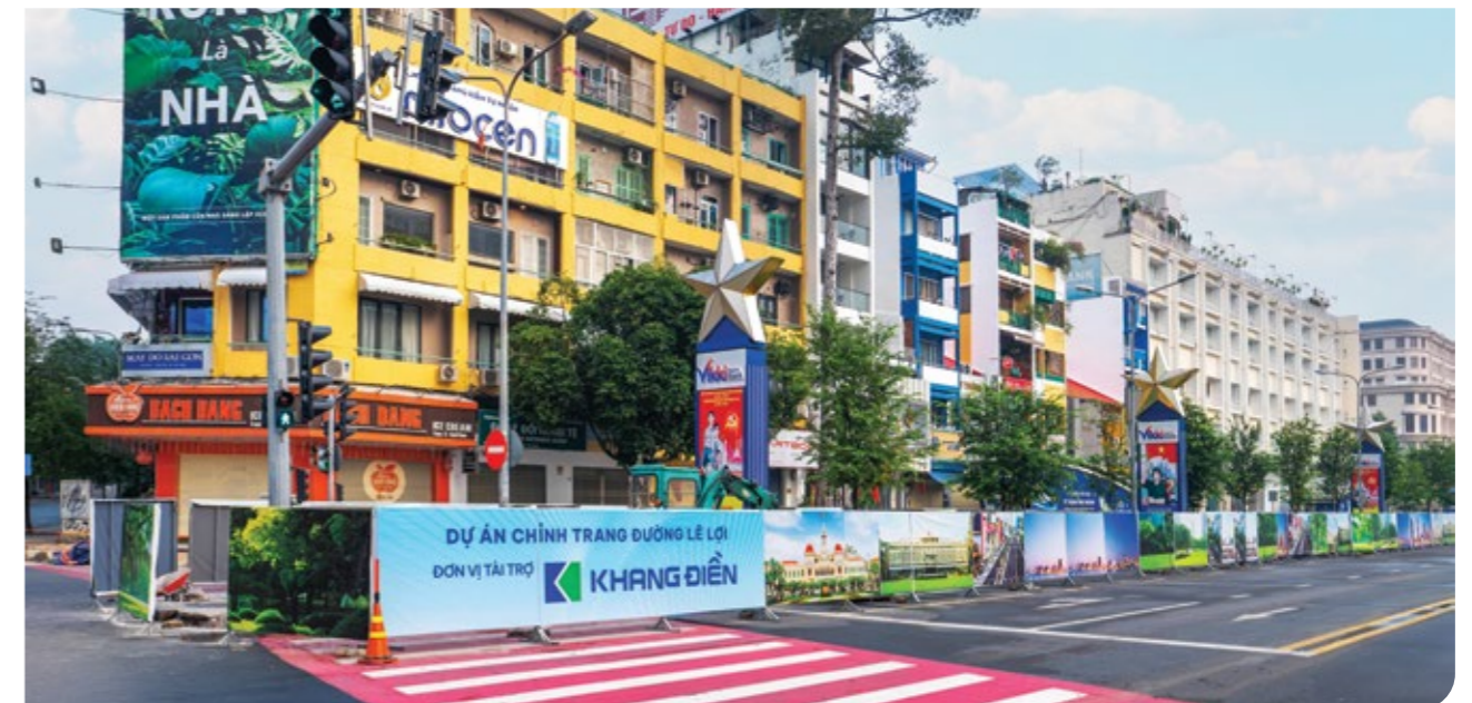
Le Loi Street Renovation Project.
